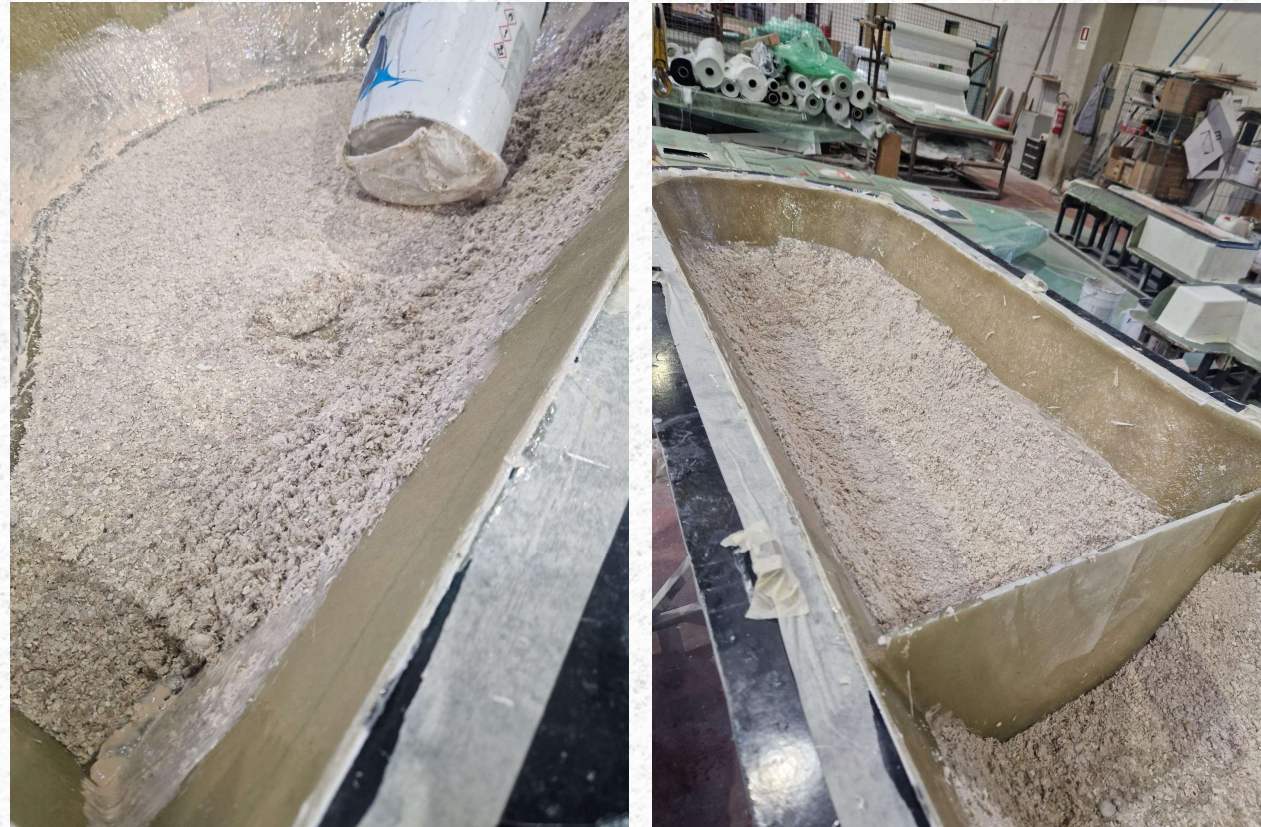
Image: Application of GFRC mixture
